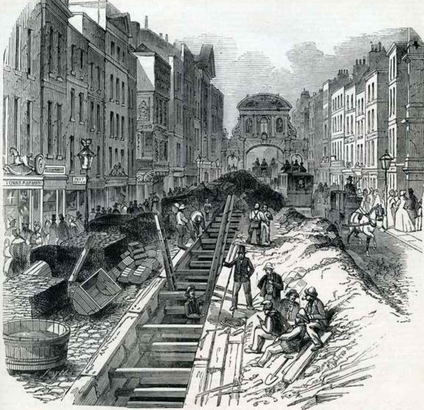
FLEET-STREET,—DEEPENING THE SEWER.
